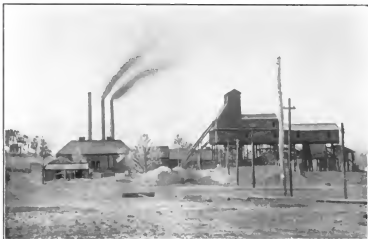
TIPPLE AND POWER HOUSE, BLACK DIAMOND MINE, DRAKESBORO.
